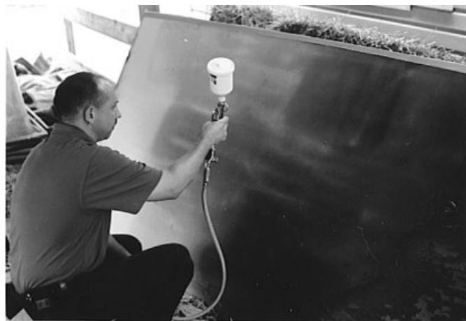
FIG. 1—Spraying liquid latex onto heavily sooted wallboard.
